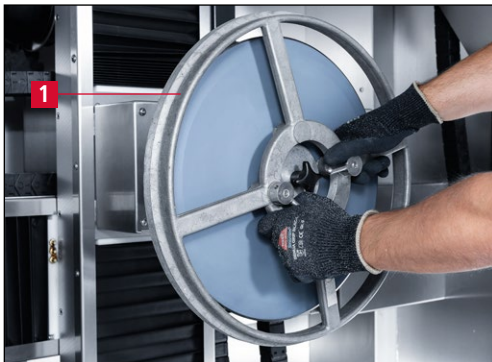
Figure 7-49 Removing the knife protector
