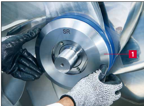
Figure 5-10 Installing the end ring (SR)
